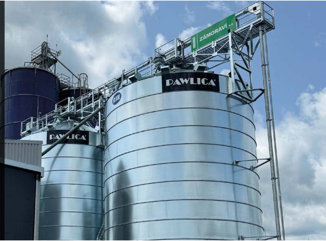
Construction Process of BIN Silos NBIN500W – 2 units, each with a capacity of 805 m 3 .
