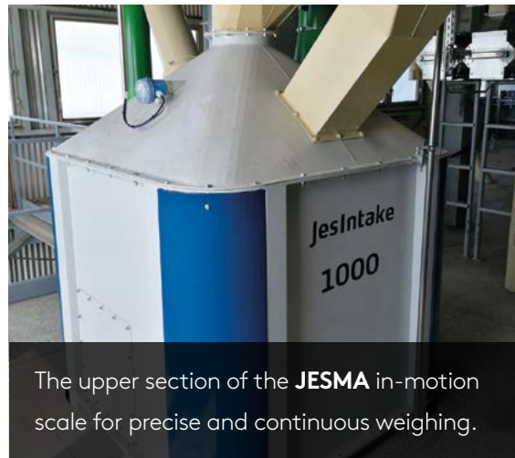
A delegation from our supplier, the Swedish conveyor company Skandia Elevator, visited to inspect the ongoing project. Their conveyors—elevators and redlers—are a key component of this demanding yet highly important modernization.
